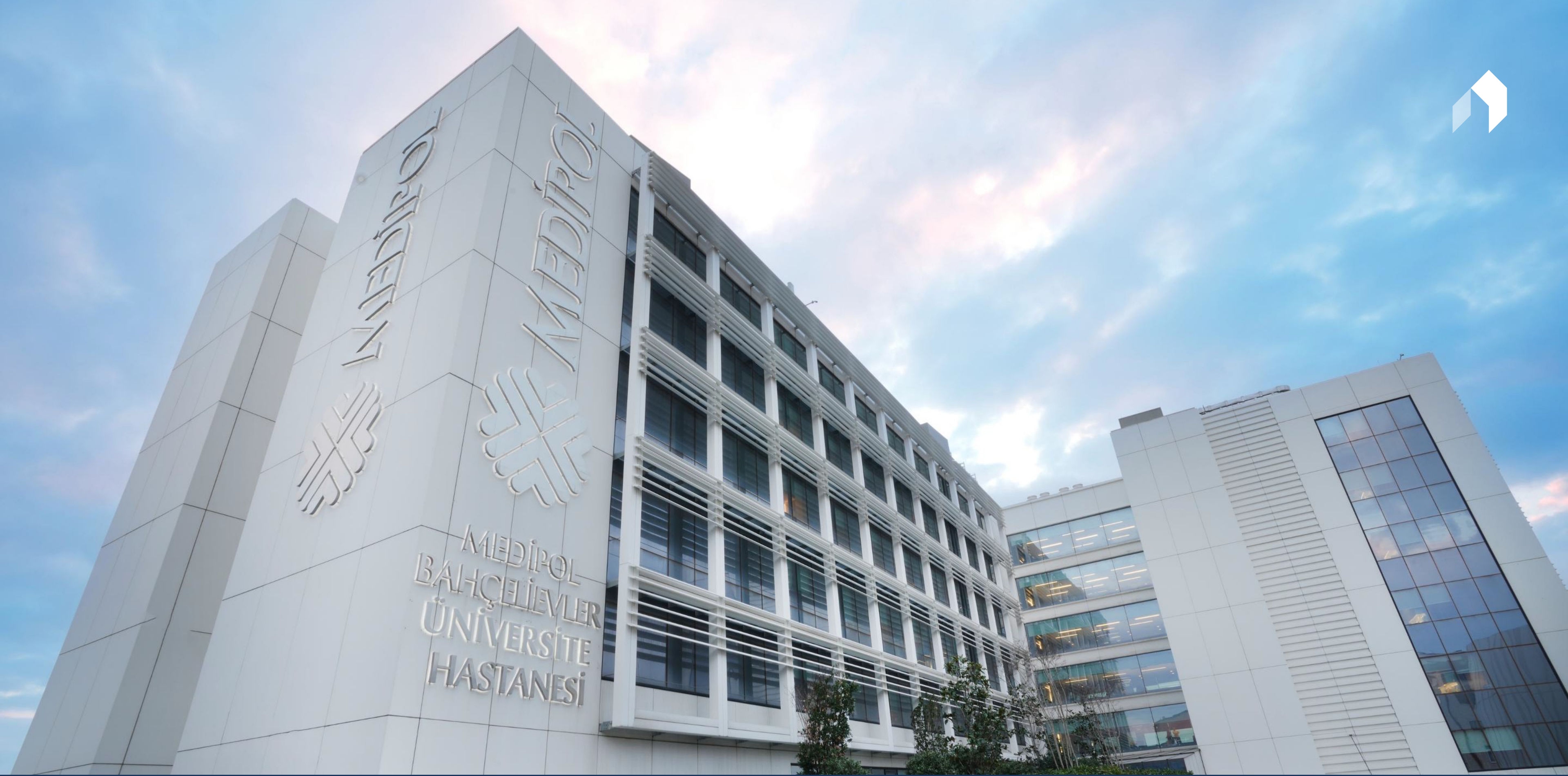
MEDIPOL BAĞCELİEVLER KRANKENHAUS
